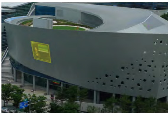
[F-2] Auditorium Outer Wall $ 10,000
